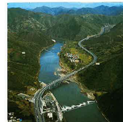
A portion of Seoul-Pusan Expressway.
