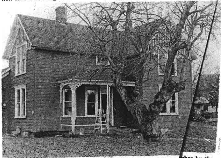
THIS LARGE four bedroom house was leased in December by the Washington County Community Action Program to serve as an emergency shelter house.
