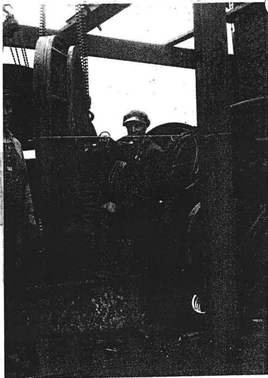
#19a & 19b. 1942. Lee Johnson, donkey doctor at Consolidated Timber Co. It appears that the donkey was burned in a fire. Lee lists this as a 13 X 14 Willamette two-speed yarder s#2482. 225 lb working pressure 72" boiler with 2" tubes X 8' long. Fire box = 7' X 5 X 4.' Westinghouse air compressor supplied air controls except to strawline drum. The engines were faster and had more line capacity than the 12 X 14. 7/8" haulback, 1 1/2" mainline. the main-line drum barke = 6' in diameter, and was located on the left side of the drum. This type had 1 1/2" injectors on each side and represented the latest and best of Willamette Iron & Steel Works.
